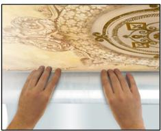
5. Unroll around 50 cm of fresco's canvas taking off a polyethylene film and hang it to the ceiling. Hold a tube with a fresco as close as possible to the ceiling.
