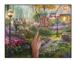
6. In the center of joints make a curvy line with a metal paint edger or broad knife cutting 2 strips at the same time. Change the blade on your knife very often for better results.
