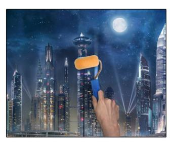
3. Carefully smooth the joint with a thin roller.
