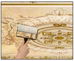
Glue the fresco unrolling the roll little by little and pressing out the excess of the adhesive and air.
