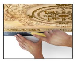
Trim away excess using a sharp knife and a liner as a guide. Change the blade on your knife every strip for better results.
