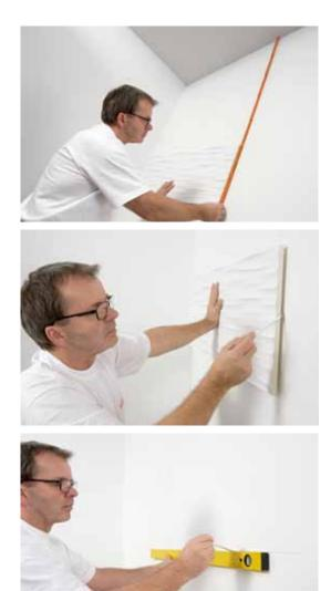
Measure out the wall and establish the position of the individual panels using the spirit level.
