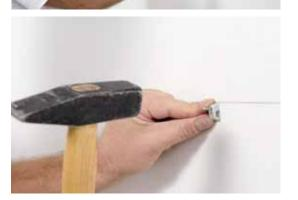
On the lower laying line, use nails and wooden battens if necessary or nail clamps.
