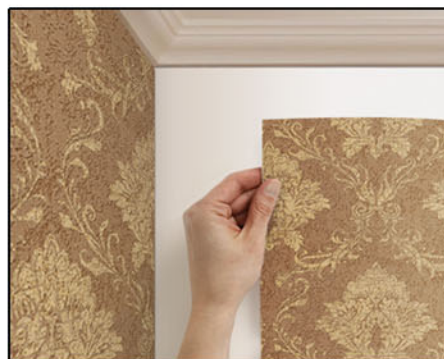
5. Strips have to be joined strictly in the corner between walls with an overlap of 3-5 cm.
