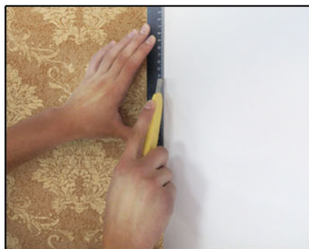
4. Trim away excess using a sharp knife and a liner as a guide. Change the blade on your knife every strip for better results.
