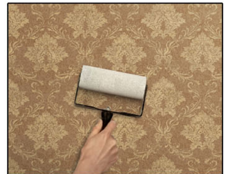
3. Carefully push any bubbles and wrinkles out toward the borders with a paint-roller.
