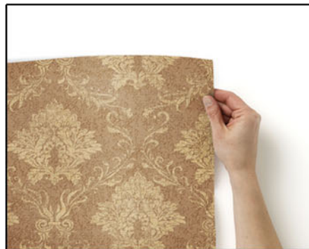
2. Apply the wallpaper adhesive to the wall and hang the canvas to the wall.
